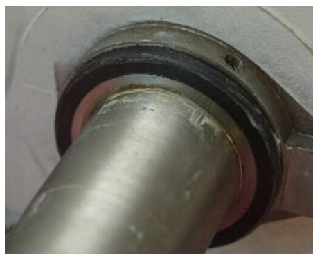
With the RA worm gear removed a fair amount of corrosion was observed on the RA spindle along with some rough machining. Its doesn't show well in the photograph above
